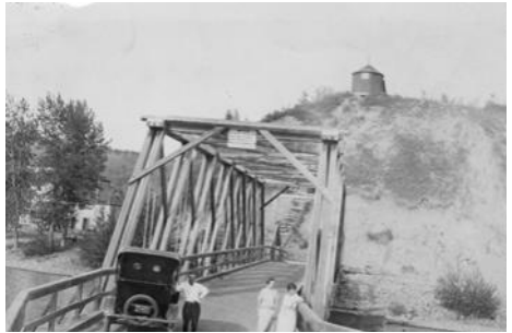
Bulkley River Bridge
