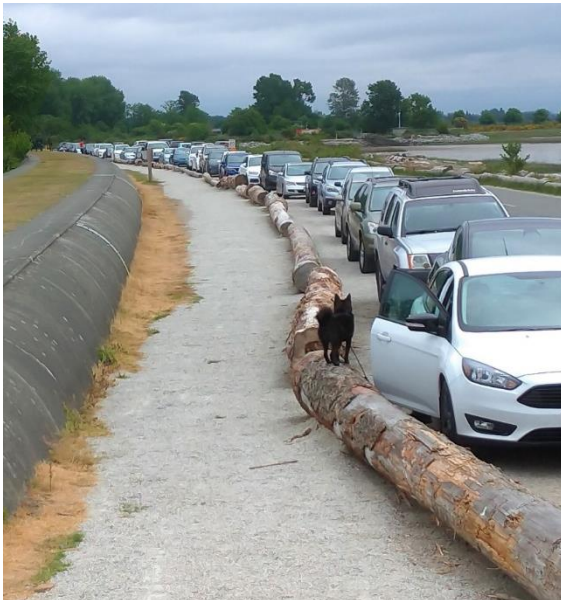
Iona Beach in Richmond, BC recently converted angled parking to parallel parking and added walkway separated by a row of logs sourced from a local beach to separate vehicles and active transportation users
