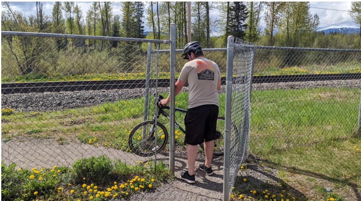
There is a corral next to the rail crossing that makes it difficult for cyclists to use the route. Modern BC AT Design Guide standards recommend against such a treatment.
