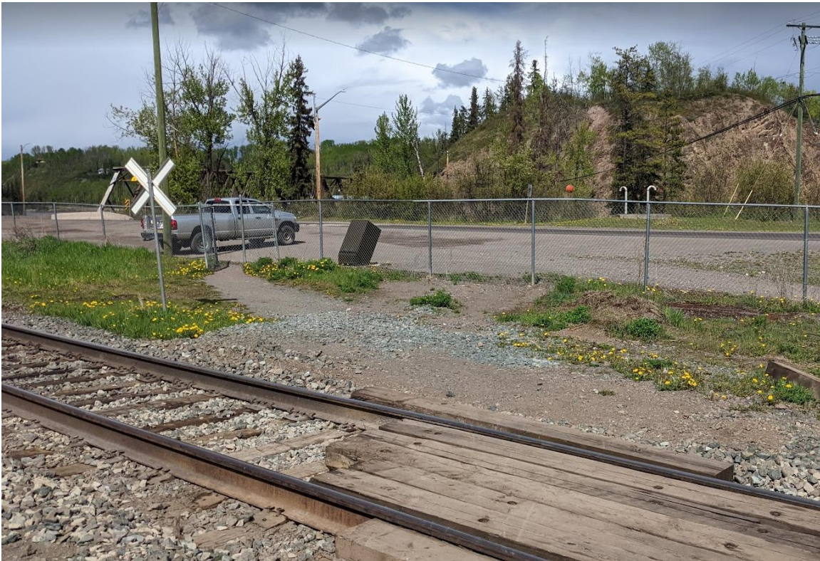
Existing active transportation rail crossing looking north towards Bulkley River bridge. The crossing does not have a perpendicular crossing angle, smooth rolling surface, or indicator warning lights.
