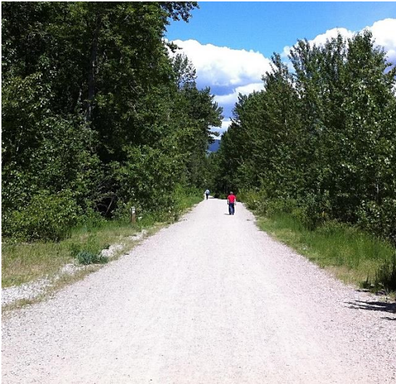
Cartpath gravel forms a hard surface that is suitable for active transportation. 3/8in Cartpath material example shown on the Mission Creek Greenway in Kelowna BC. Images Retrieved from: https://www.hikinqaddiction.ca/trails/viewtrail.php?trail_id=11 &
