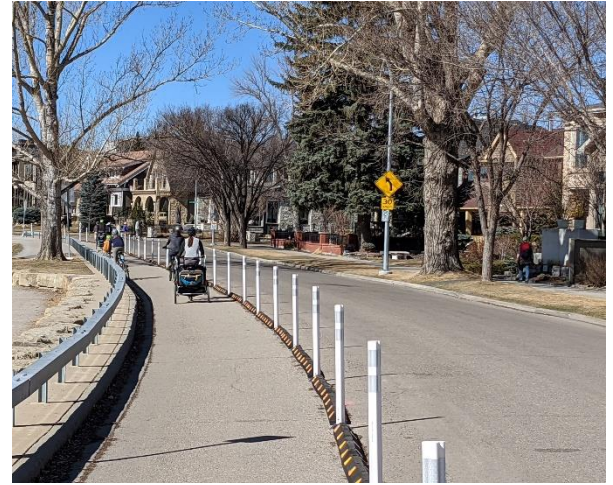
Example of a quick-build MUP in Calgary, AB using rubber barrier curb and plastic delineators
