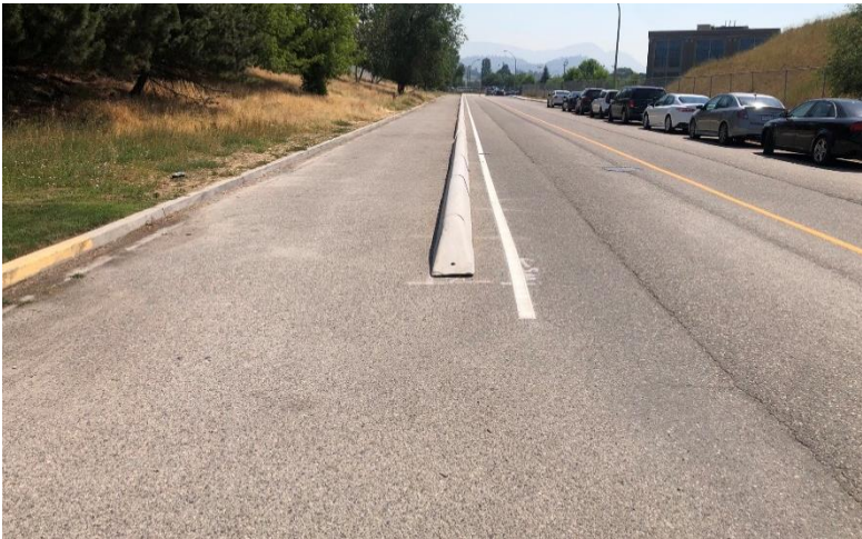
Example of a quick-build MUP in Kelowna, BC using line painting and pre-cast concrete barriers
