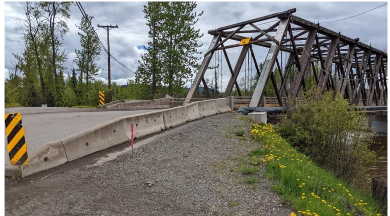
The current approach on the north side has no pedestrian accommodations to crossover to the bridge's walkway.
