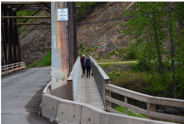
The bridge's walkway is narrow but separate from vehicle traffic. The narrow width makes it difficult for cyclists to use it if there are others on the bridge.
