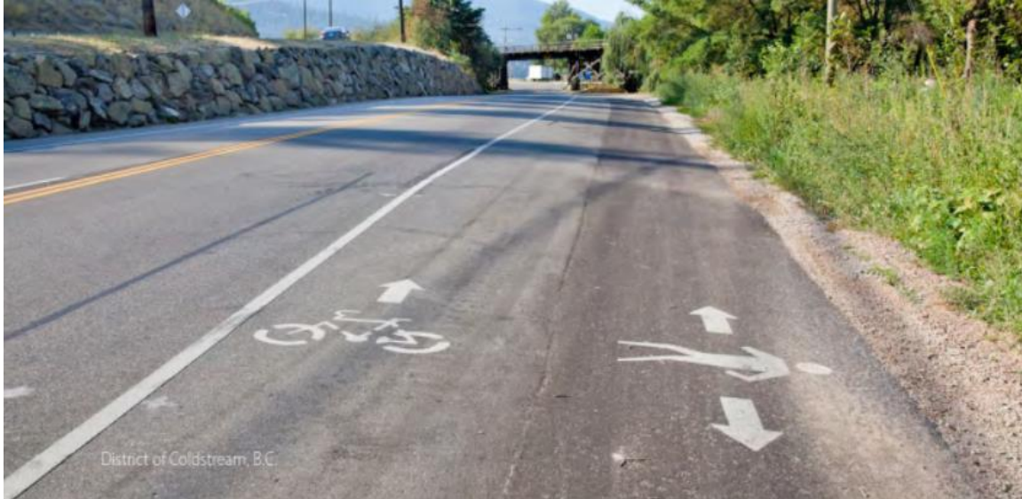
Example of a walkable shoulder in Coldstream, BC. Image Retrieved From: BC AT Design Guide
